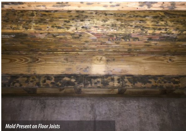
Mold Present on Floor Joists
