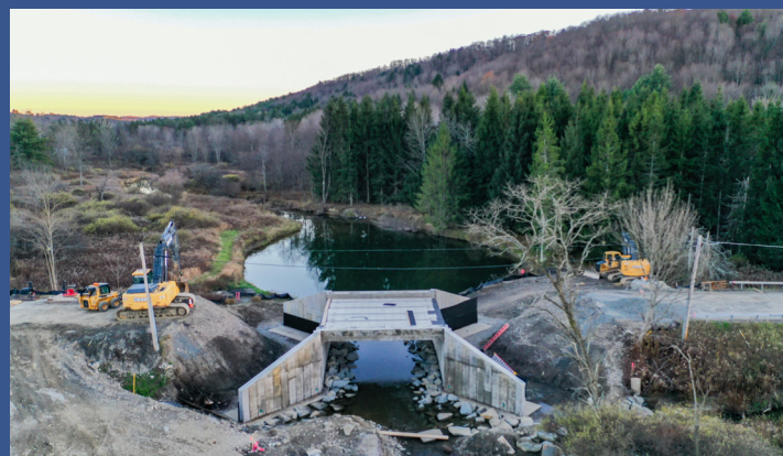
Above: Dutchtown Road Three-Sided Culvert
