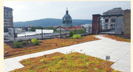
73 Court St. Green Roof - Binghamton, NY
