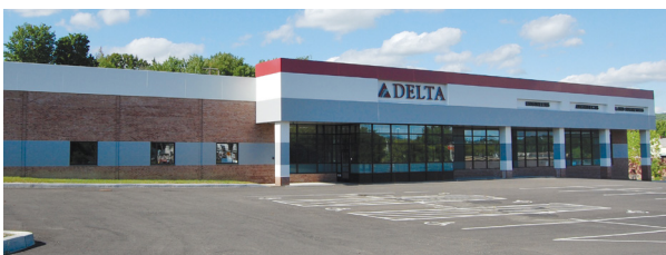
Delta Corporate Office in Endwell, NY - a LEED Gold Facility
