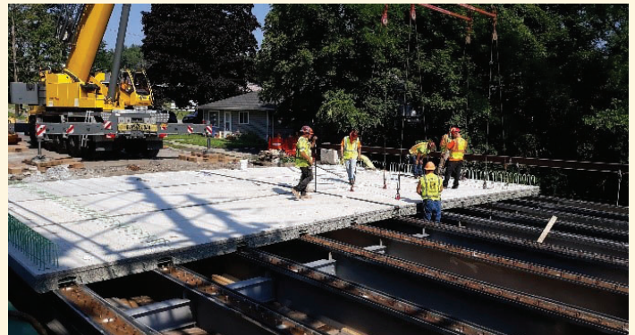
ABC Precast Deck Panel Installation
